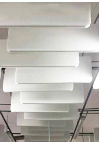
JustFiber Baffles sound-absorbing baffles panels have been designed to be inserted in wide environments and are intended for large-scale installations in gyms, swimming pools, school canteens, schools, collective spaces or industrial premises. The sound-absorbing baffles allow a very efficient acoustic correction intervention with high acoustic performance (sound absorption class "A") and at the same time guarantee the requisites of effectiveness and economy for their quality / price ratio.
